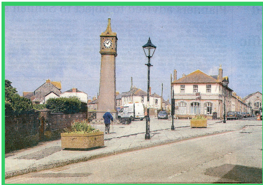
Above: Bank Square after the cables were removed and located underground
